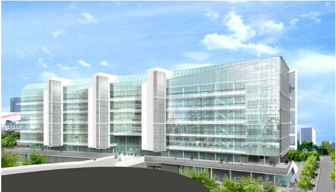
Trading Floor building at La Défense. Copyright : Ateliers 234
